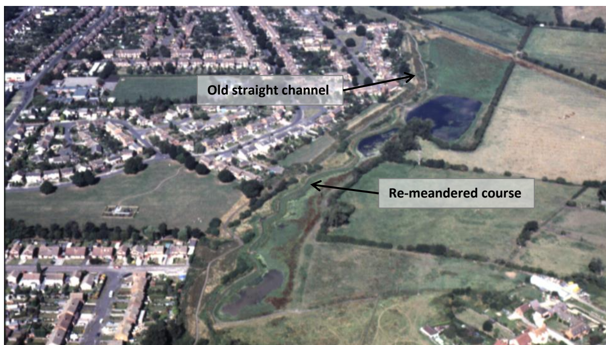
Aerial view of the Brook and flood storage/overspill area
