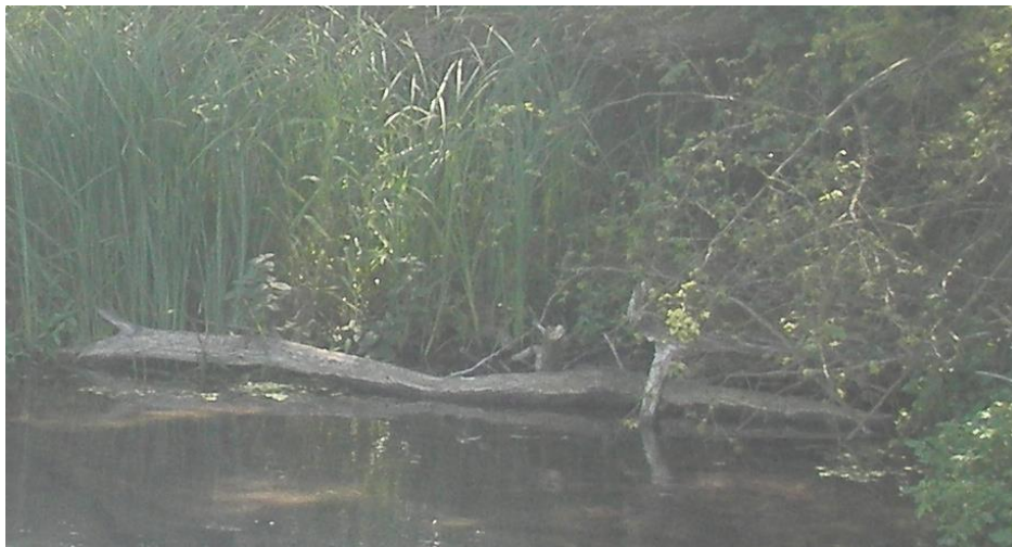
Example of the use of woody debris – note dimensions and level would need to be adapted for the specific site
