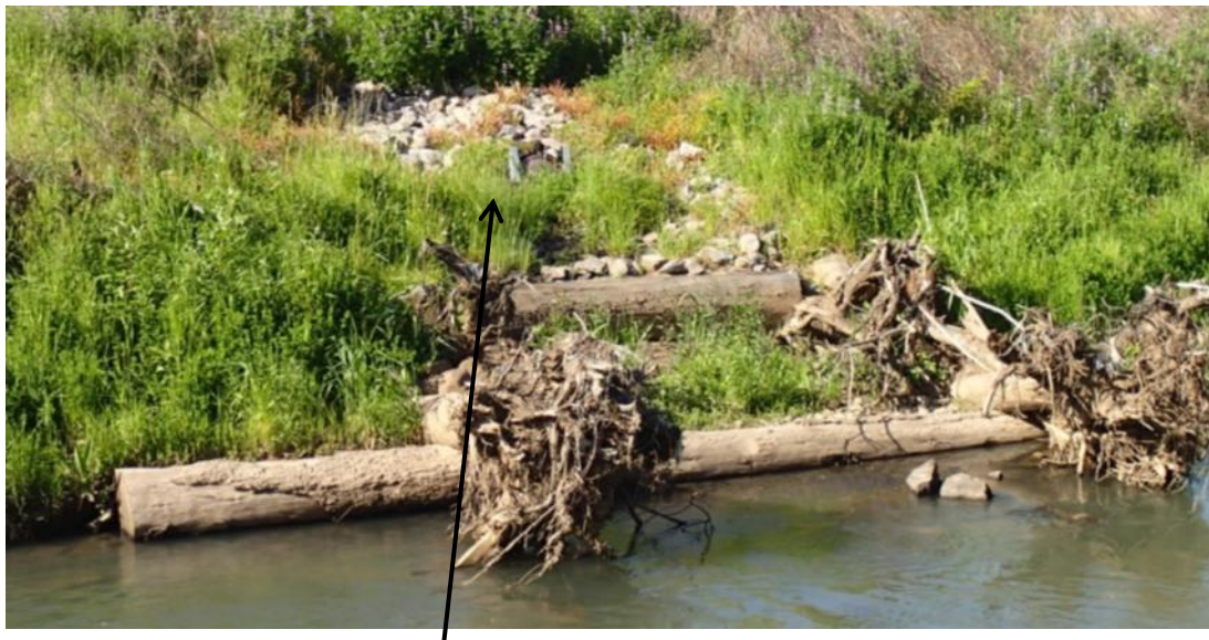
Outfall setback with vegetation, gravel and staked in wood for habitat
