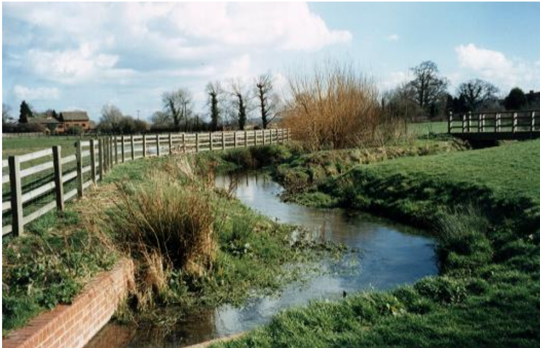
Four years on and vegetation is shaping the low flow channel, establishing in the deposited silty margins
