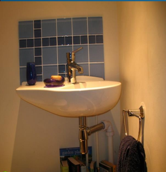
Sink on wall with no vanity unit
