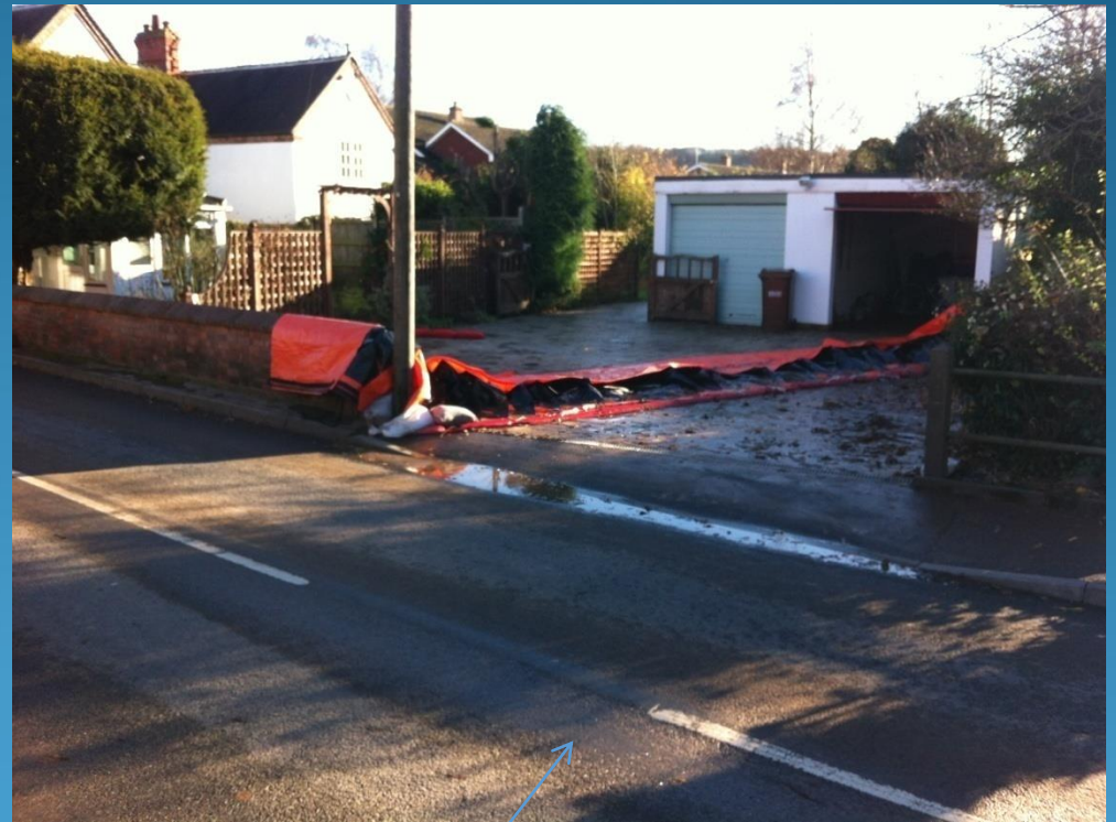
Post flood photo
