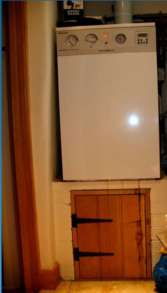
Boiler raised up
