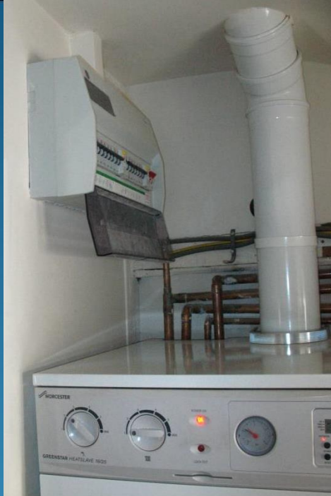
Fuse box high up
